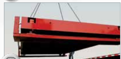
2 Unload and set modules.
