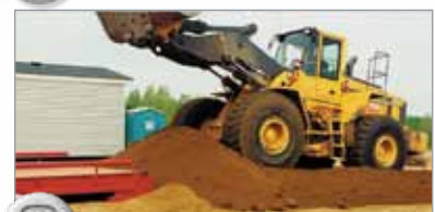
3 Backfill to bulkheads and finish ramps.
